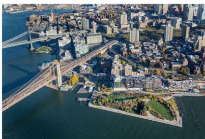
Brooklyn view looking across from Pier 5, Brooklyn Bridge Park (Photo: Through a complex urban context)
